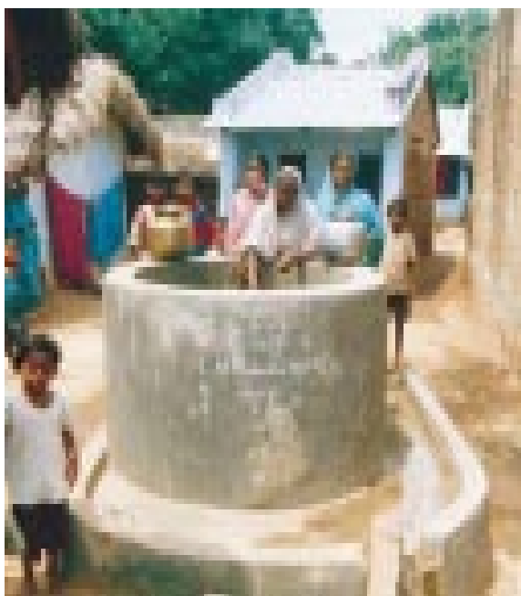
A Drinking water well constructed under JGSY
