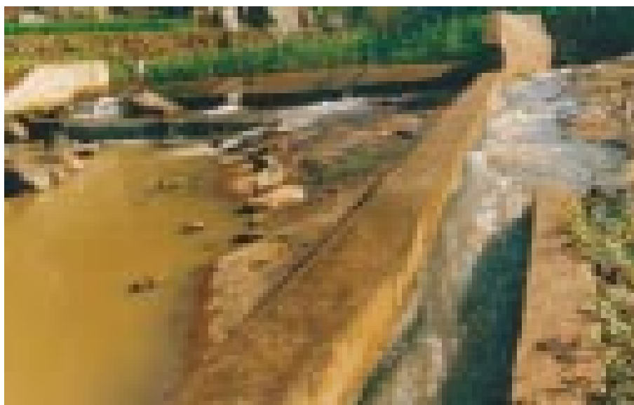
Construction of Minor Irrigation Project under EAS
