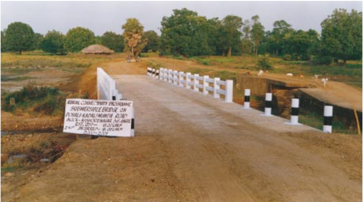
Depicting submersible bridge constructed under PMGSY to provide connectivity
