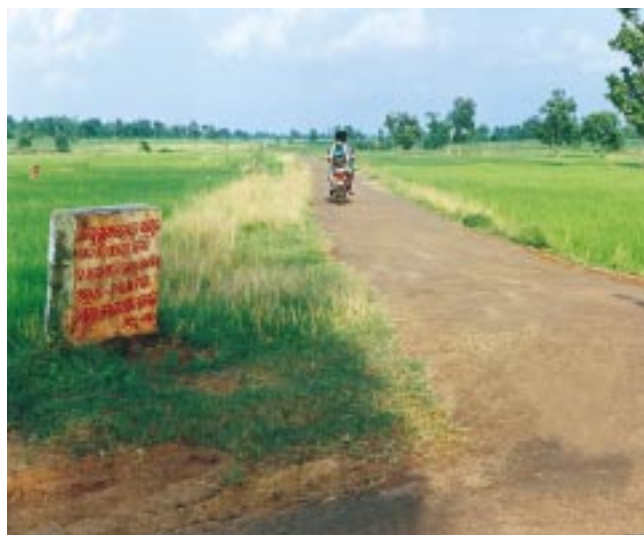
Road Constructed under Pradhan Mantri Gram Sadak Yojana
